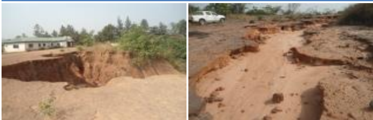
Figure 1: Show severities of the collapsed roads 1
